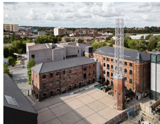
/Project: Rutland Mills – Wakefield, Yorkshire
